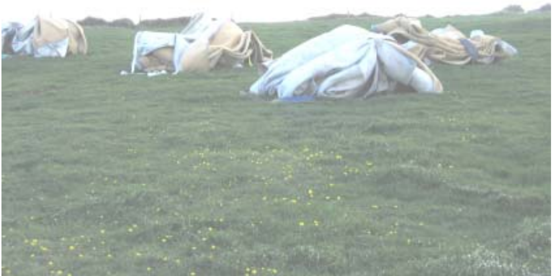
Photograph 1 Geo-textile bags awaiting deployment
